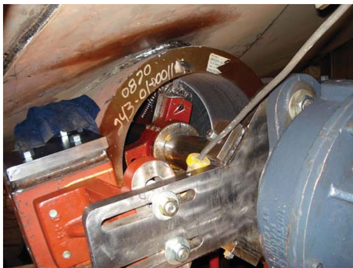
On-site rudder tube machining with MBMC4 Boring System positioned vertically
