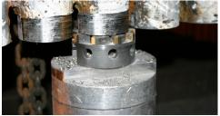
Overlay is removed from new and existing tubes and their ends are prepared for welding to new tubes
