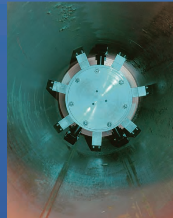
Pipeline clamp in 24" Sched 40 pipe
